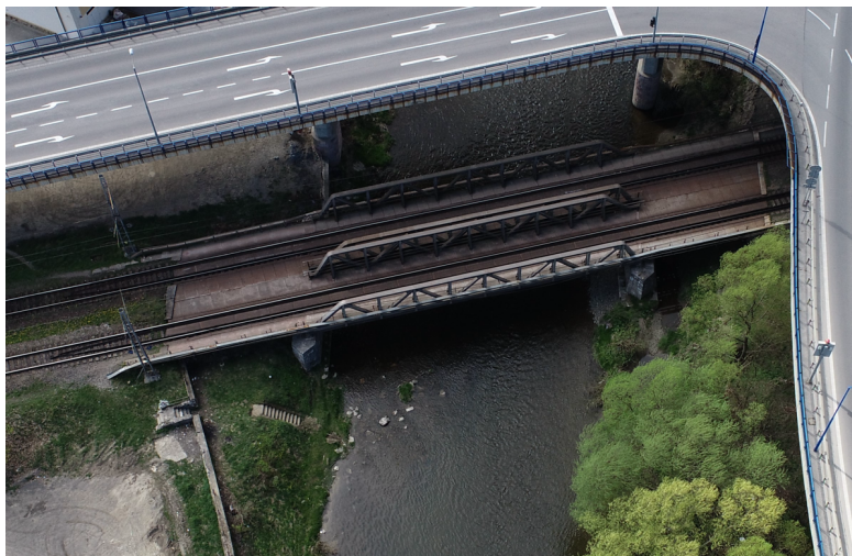
Figure 1 Case study railway bridge
