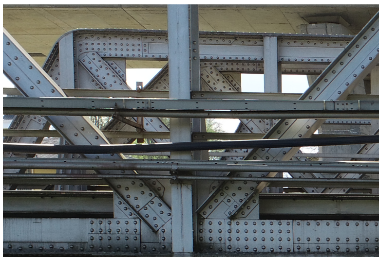
Figure 2 Detailed look of railway bridge construction
